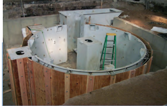
Installation of the optional steel pit foundation shell utilizing a right-hand-turn pit access stairway. Use of the shell reduces custom formwork and installation expense.
